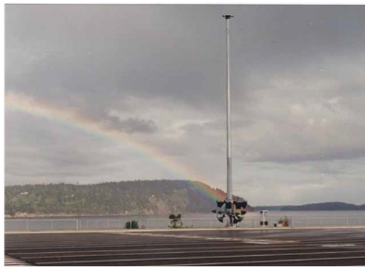
The Community Professional Loudspeakers installation at the Duke Point Ferry Terminal at Nanaimo on Vancouver Island has been facing the full force of coastal weather 365 days a year for 15 years. The cluster system, which utilizes Community's M4 compression driver on five PC1542M and three PC1564M long-throw, patterncontrol horns, was designed by MC Squared System Design Group and installed by Sound Source and Lightrix.
